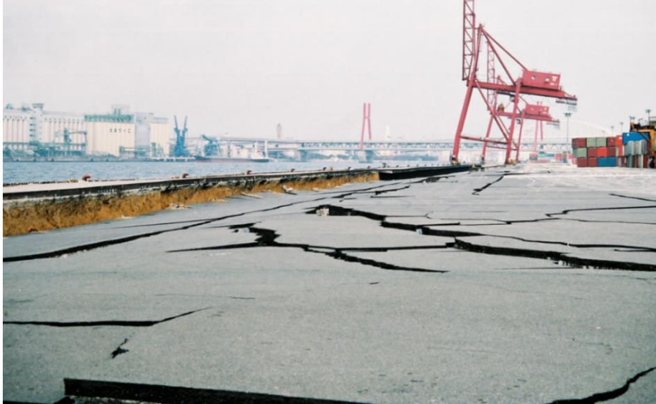
Damage to caisson quay wall during 1995 Hyogoken-Nambu earthquake
